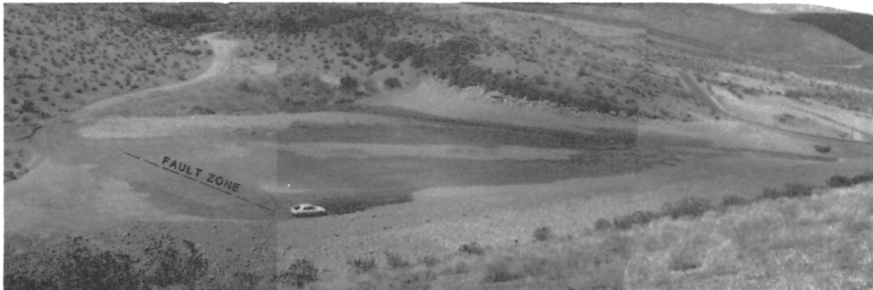
Figure 12. Area C completed. Nuisance surface flow exists along what could be a fault zone. Seepage expanded downstream in a linear fashion along this line.
