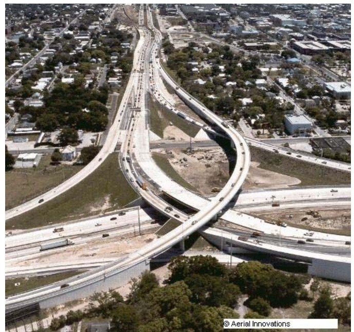
Fig. 1. Downtown Tampa Interchange bridge construction.
