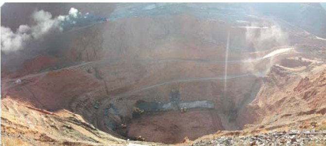
Fig. 6: Foundation excavation pictures at start, middle and end of excavation.
