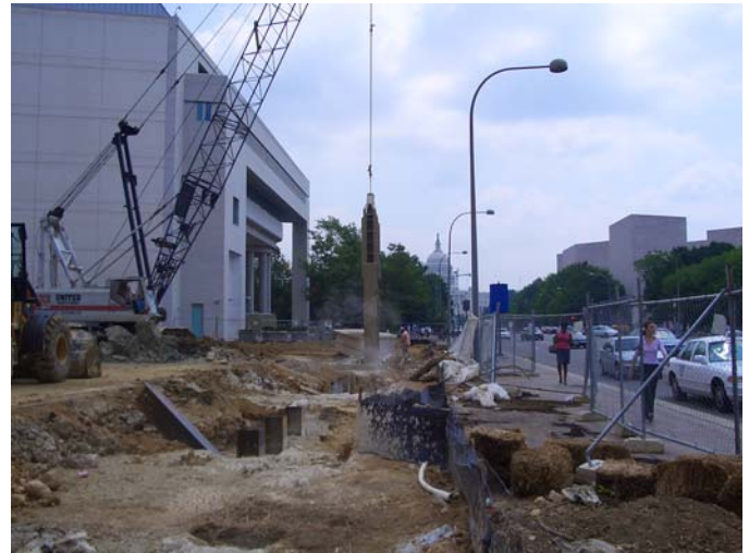
Fig. 5. Clamming operation for PSHG wall.
