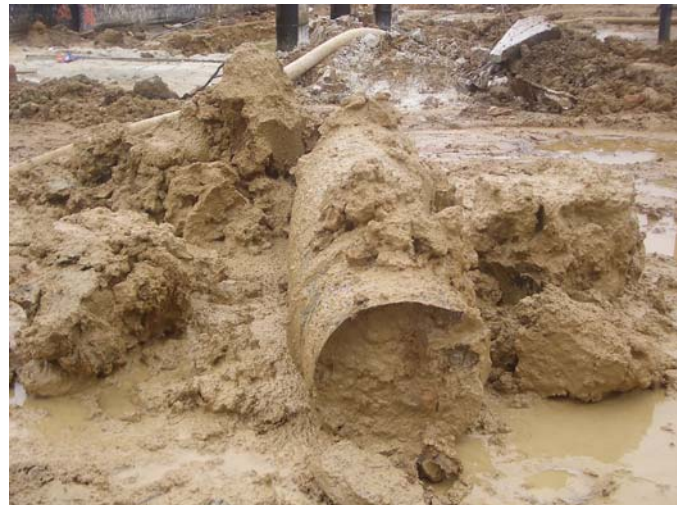
Fig. 3. Raymond Step Taper Piles removed with clam bucket.
