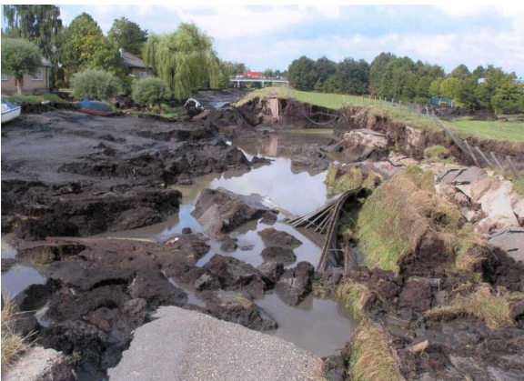
Fig. 1. Canal (left) and dike(right)
