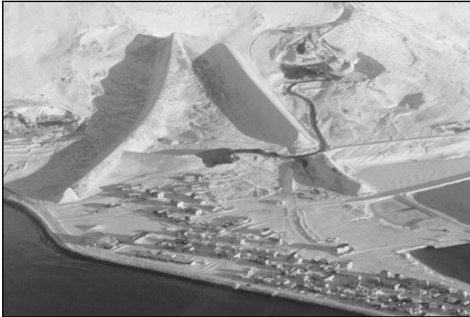
Fig. 5. A view of Flateyri during dikes' construction.
