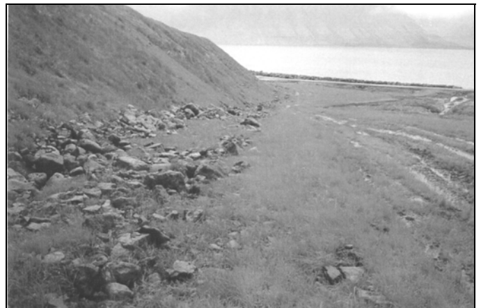
Fig. 8. Side view of downslope outer dike, note dam toe.
