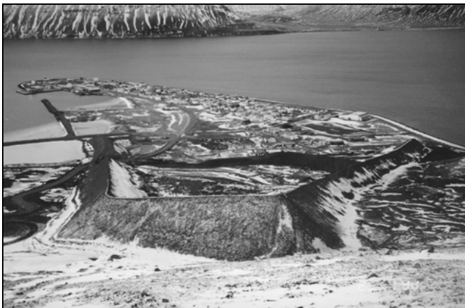
Fig. 6. A view of Flateyri with the defences near completion.
