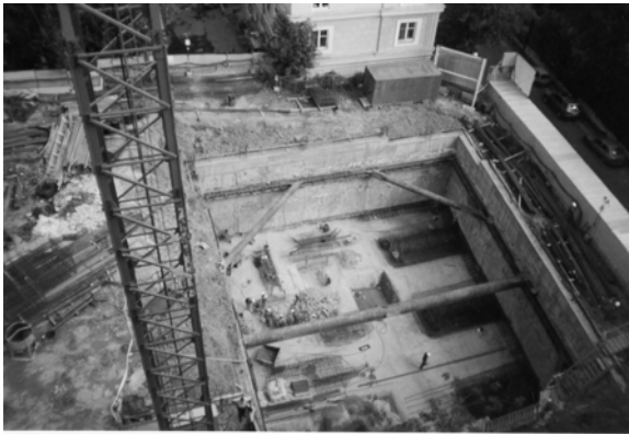
Figure 2. Foundation trench in Kapranov lane, Moscow.
