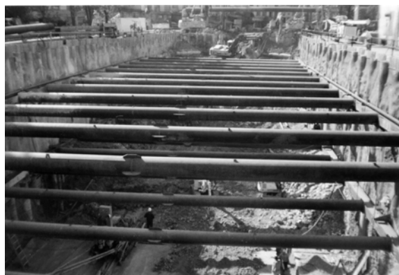
Figure 1. Foundation trench of Lefortovo tunnel.
