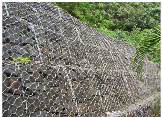
Fig.1 Gabion box made of Hexagonal double twisted wire mesh (Maccaferri)
