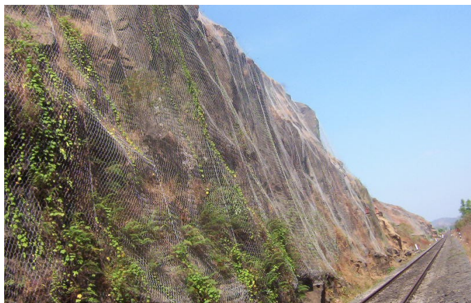
Fig.2 Rockfall netting along Konkan Railway route
