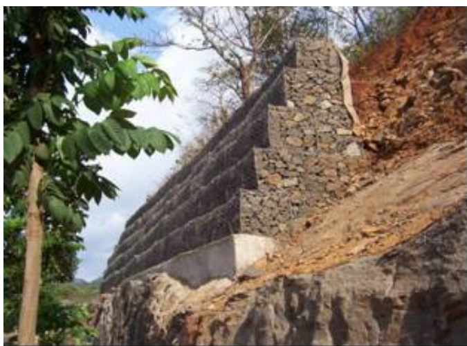
Fig.11 Gabion wall on PCC foundation for undulating rock strata, AVSLC project.
