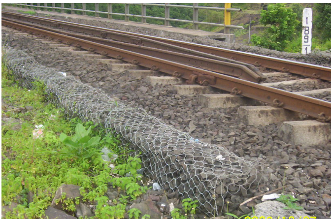
Fig.5 Baby Gabions fro ballast retention along Konkan Railway route
