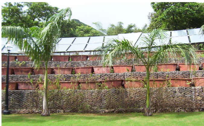
Fig.12 Gabion wall in club house area, AVSLC project.
