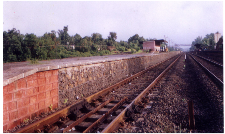
Fig.6 Platform Gabions at Kudal Railway station along Konkan Railway route
