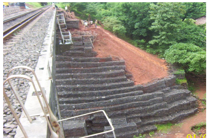
Fig.4 Gabion wall for Slope/ Embankment protection along Konkan Railway route
