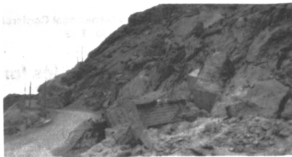
Fig.2 Rockfalls nearby the Sefid-Rud dam.
