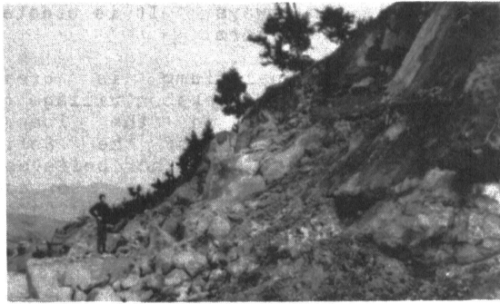
Fig.6 A planar slide in the Bareh-Sar road.
