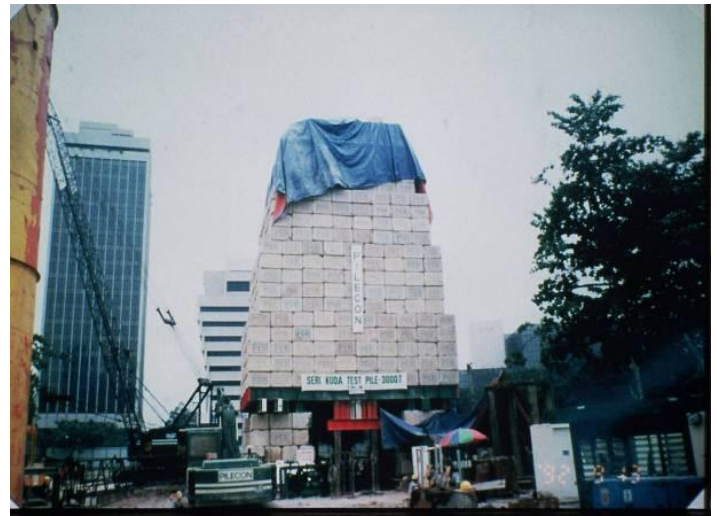
Fig. 3. 3,000 Ton Kentledge Load Test.
