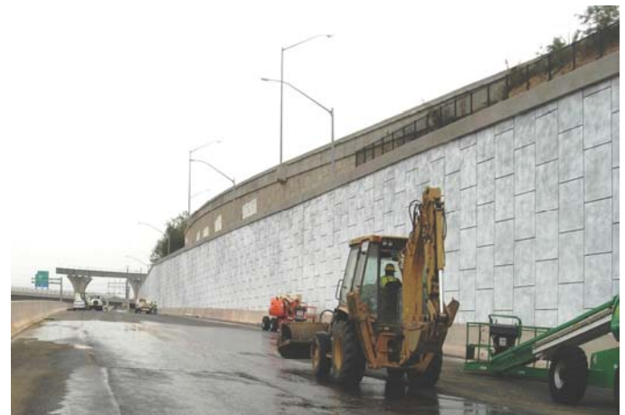
Fig. 11. Finished Wall with MSE
