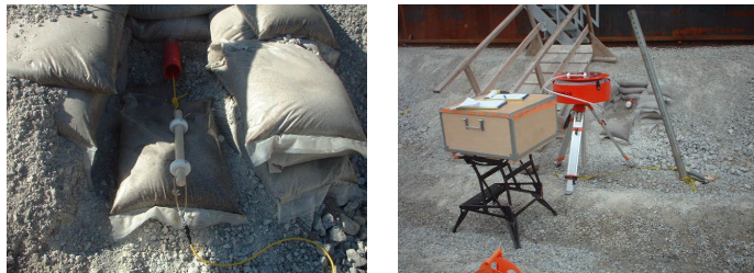
Fig. 16. PVC pipe, sensor and Consoil profiler setup
