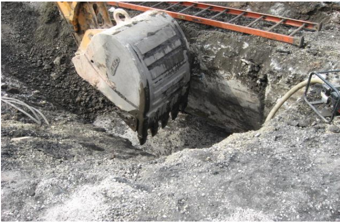
Fig.6. Excavation to Expose Pile under Pusher Track
