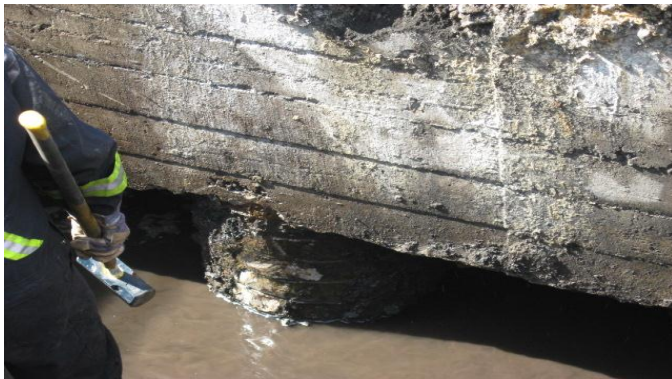
Fig.7. Located Pile under North Side of Pusher Track
