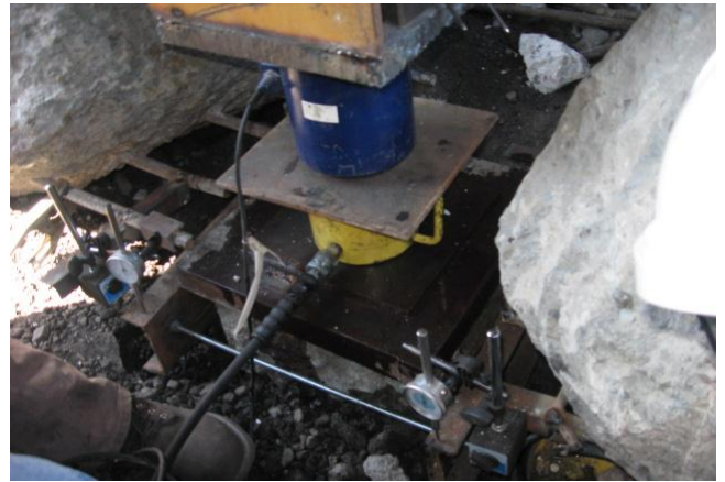
Fig. 8. Test Set Up For Pile Load Test
