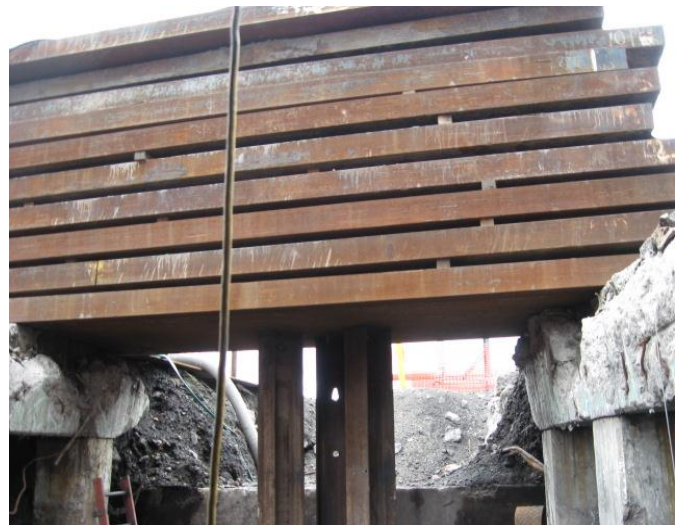
Fig.10. Reaction Weights- Steel Slabs
