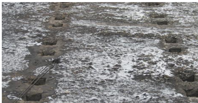
Fig.1. Existing Surface of Oven Pad - No. 6 Coke Battery
