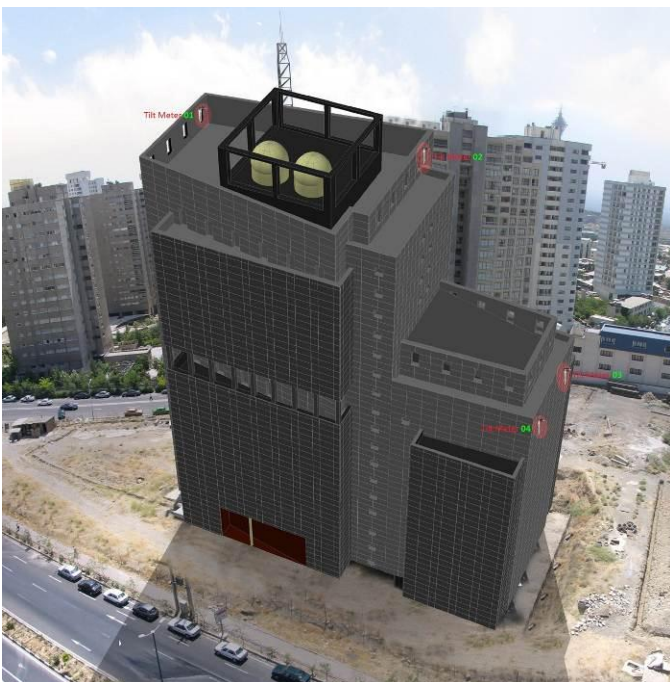
Fig. 2. 3D view of the building and the location of the tilt meters
