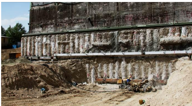
Fig. 11. Excavation of block 7 during the 2nd lift of excavation
