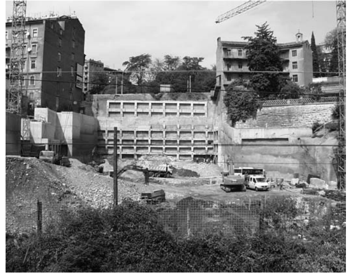
Fig. 3. A view of the open pit during the execution
