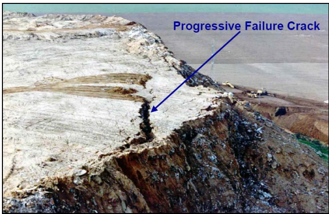
Fig.7. Top of Hiriya landfill after slope movement (Isenberg 2003)
