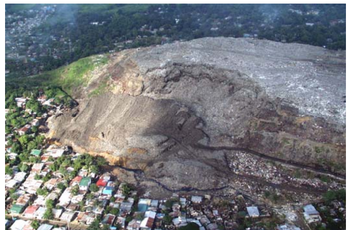
Fig. 9. Payatas landfill slope failure in 2000. (Kolsch and Ziehmman, 2004)
