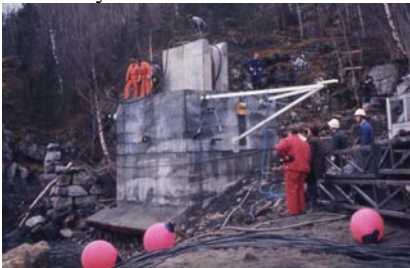
Fig. 1. Anchor block on launch skid prior to deployment
