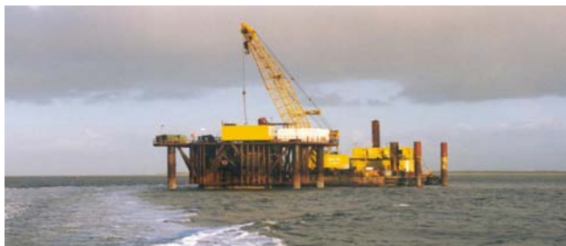
Fig. 1. Tie-in Chamber during construction
