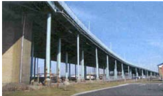
Fig.1. View of part of the bridge
