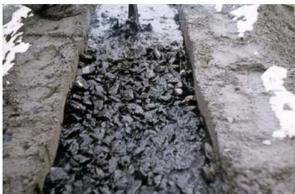
Fig. 2. Injecting hot bitumen into gravel matrix
