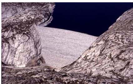
Fig.1. Photograph of Svartevann dam
