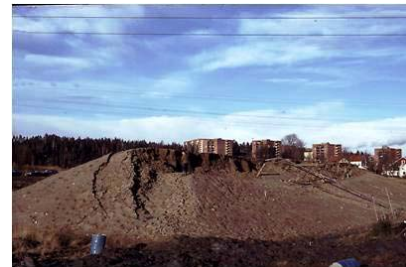
Fig. 4. Photograph after failure
