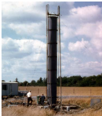
Fig.1 In situ shear device on location
