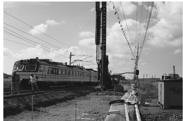
Fig. 2. Installation of lime-cement columns in Ledsgård, June 2000, Sweden, (J&W / WSP, 2000).
