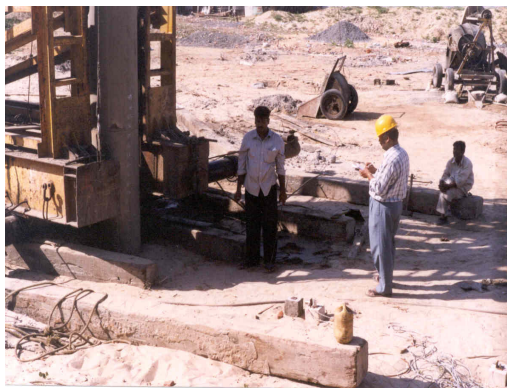
Partly driven pile
