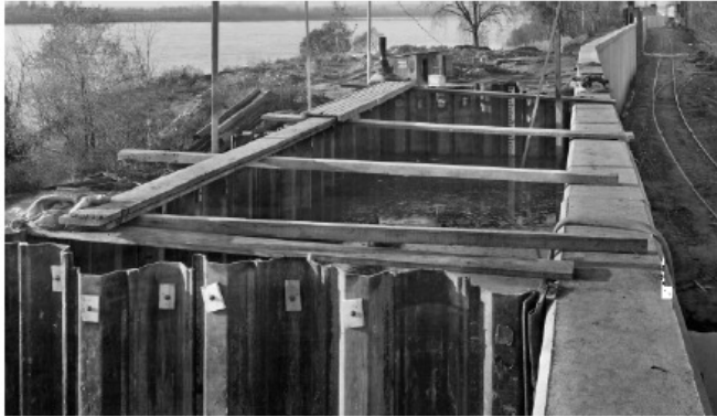
Fig. 1. Test Structure for Test Series No. III – Tell City, Indiana
