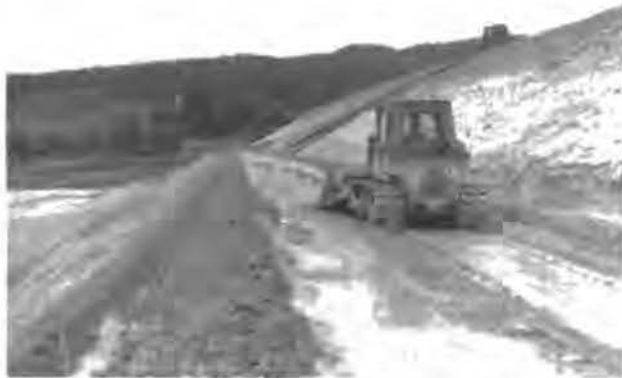
Fig. 7 Dozer Compaction in Narrow Construction Cell - L-L Dam (1983)
