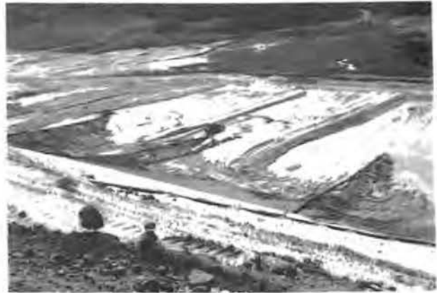
Fig. 6 Downstream Berm Construction - L-L Dam (1982)
