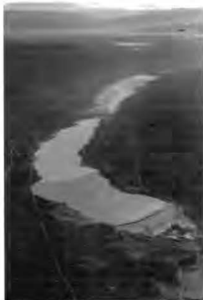
Fig. 1 Lornex Tailings Disposal Facility (1983) (From Background: H-H, J-J and L-L Dams)
