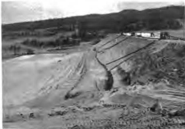
Fig. 5 Downstream Shell Construction - L-L Dam (1983)
