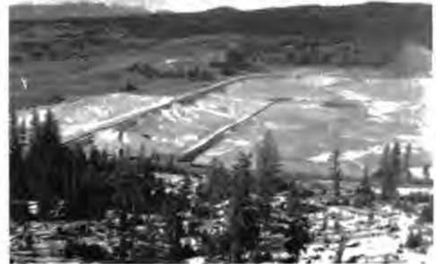
Fig. 4 Upstream Shell Construction - L-L Dam (1983)
