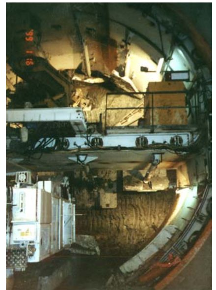
Fig 7. Face of the shield machine
