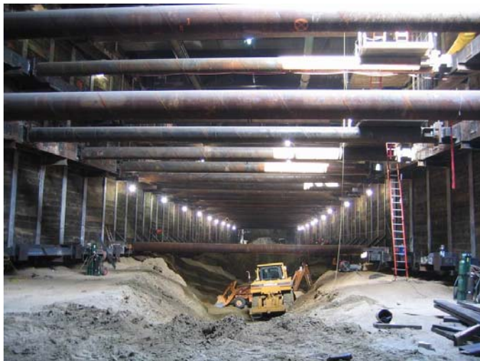
Fig. 6. Notch cut prior to installation of third level of bracing
