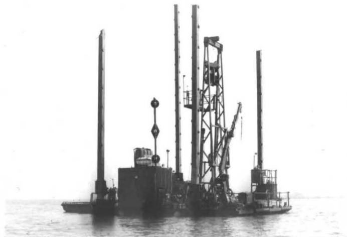
Fig. 3 General view of jack-up drilling system
