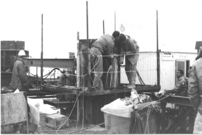
Fig. 27 General view for horizontal pile load tests
