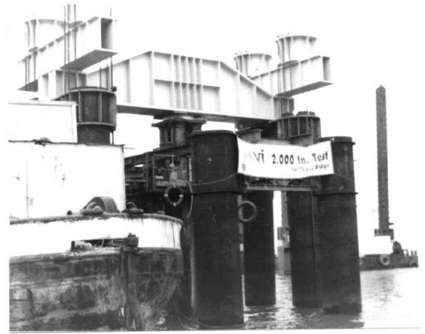
Fig. 25 General view for vertical pile load tests
