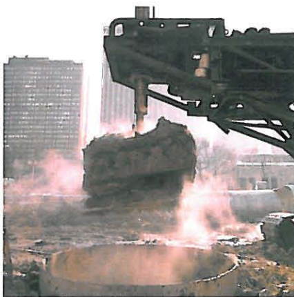
Fig. 19. Water Tower Place - large crane attachment augering 10 ft. diameter shaft (1972)
