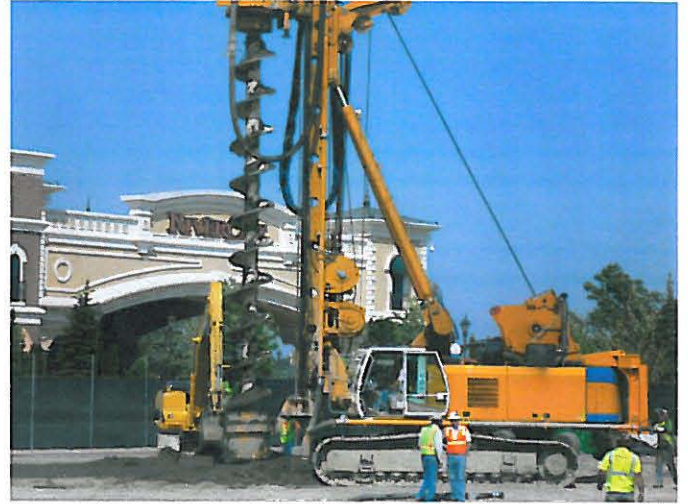
Fig. 33. Installing 48" Diameter CFA Piles to Rock. (2011)
