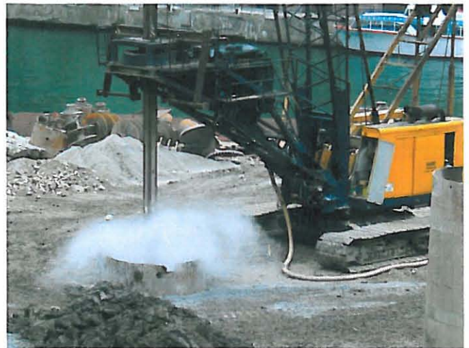
Fig. 26. Cluster Drill in use at Trump International Tower. (2005)
