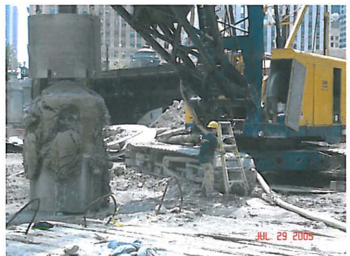
Fig. 27. Discharging cuttings from calyx basket above 60” cluster drill – Trump International Tower (2005)
