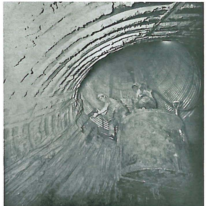
Fig. 22. Water Tower Place - hand trimming top of 27 ft. diameter bell. (1972)
