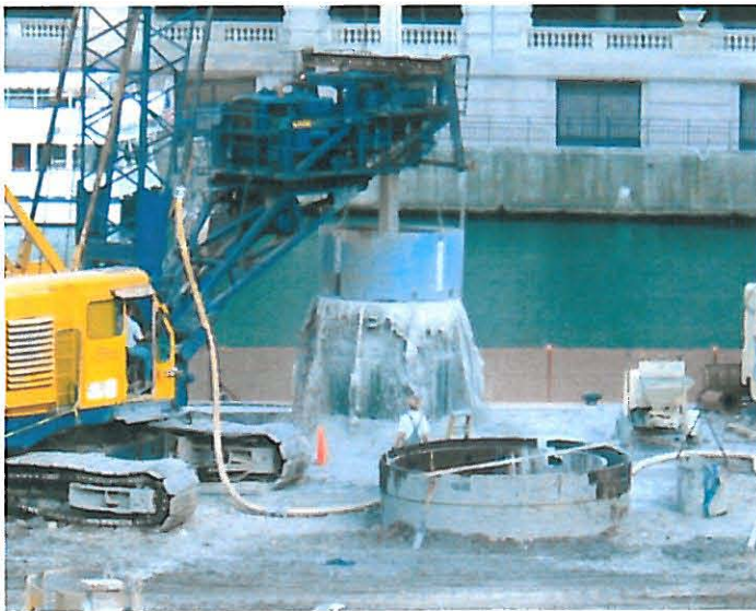
Fig. 30. Discharging cuttings from calyx basket above 114" Hole Opener - Trump International Tower (2005)
