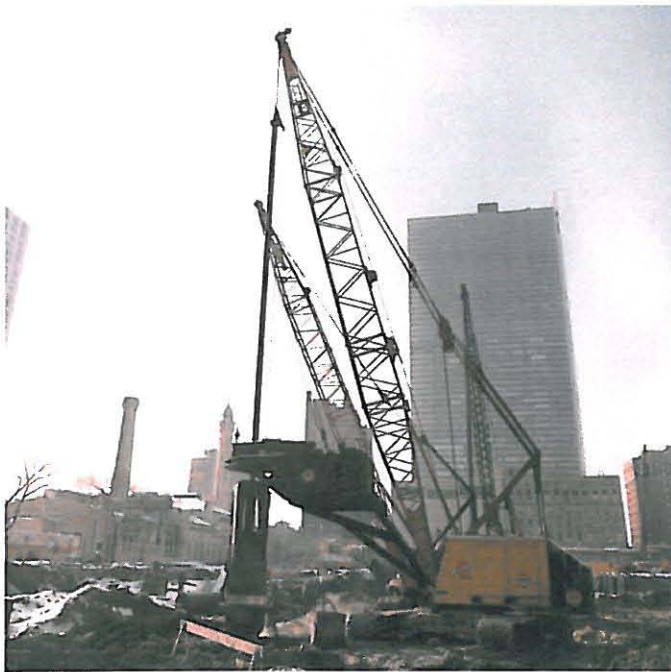
Fig. 18. Caisson Installation at Water Tower Place (1972)
