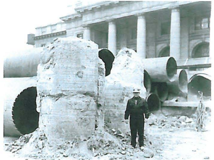
Fig. 24. Large-diameter limestone cores recovered during rock socket excavation.
