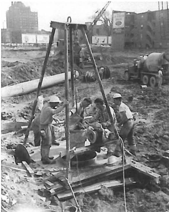
Fig. 9. Tripod Set-up with air tugger over hand-dug caisson.
