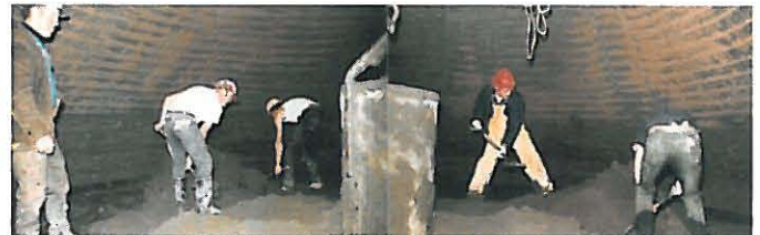
Fig. 21. Water Tower Place - hand cleaning 27 ft. bell. (1972)
