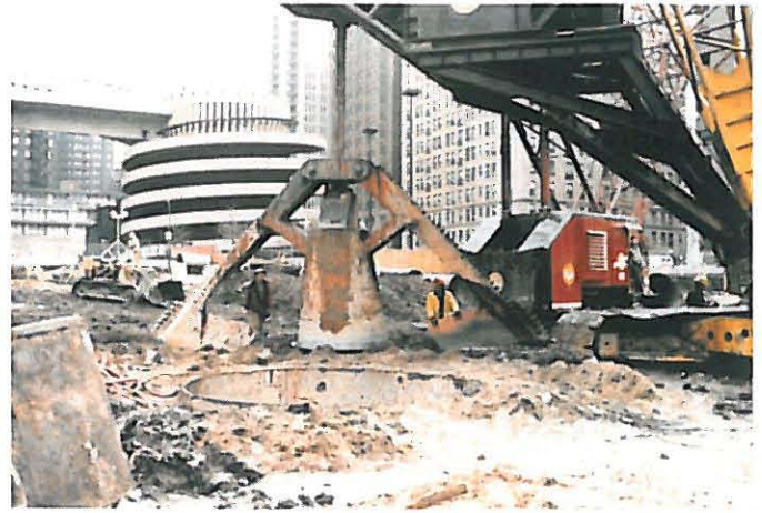
Fig.20 Water Tower Place - large "Apex" belling bucket (1972)
