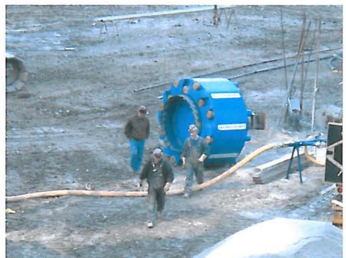
Fig. 28. 60”to 90” Hole Opener - Trump Internatinal Tower (2005)
