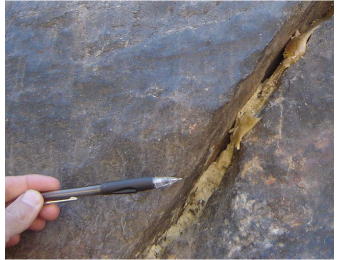
Fig. 10. Hard, dense, high-strength resin fully filling major rock mass discontinuity.
