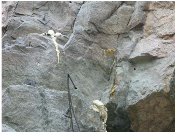
Fig. 9. Typical migration of PUR injection from below the injection point, upwards through the rock mass. Note that some of the resin is foaming due to moisture in the surface fractures.
