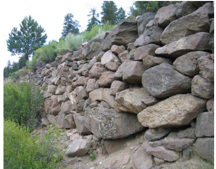
Fig. 12. Looking west along the test section.
