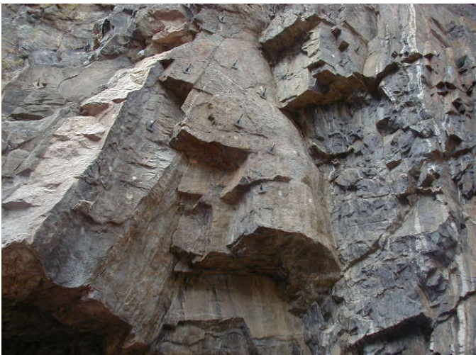
Fig. 7. Close-up of the foliation joint-defined blocks above the western portal.
