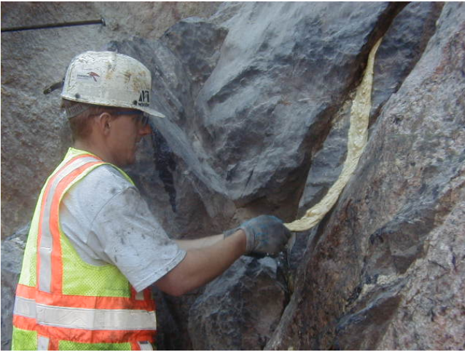
Fig. 11. Overruns are relatively easy to remove if tackled before initial set is complete.
