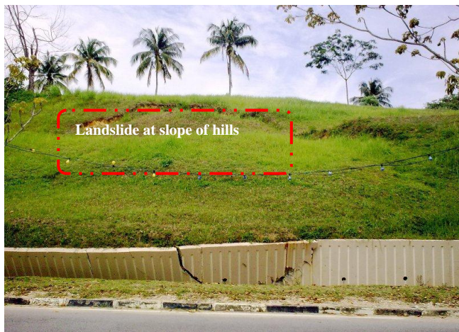
Fig.4. Landslide at UKM, Malaysia
