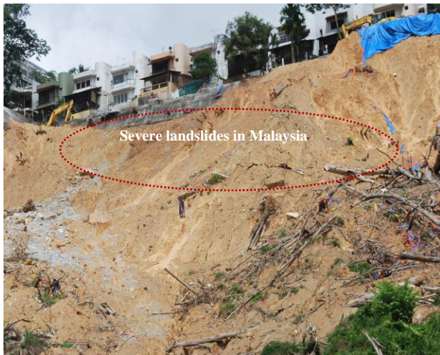
Fig.1. Landslide at Bukit Antarabangsa, Malaysia
