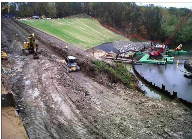
Fig. 24. Slope Grading with Temporary Working Bench
