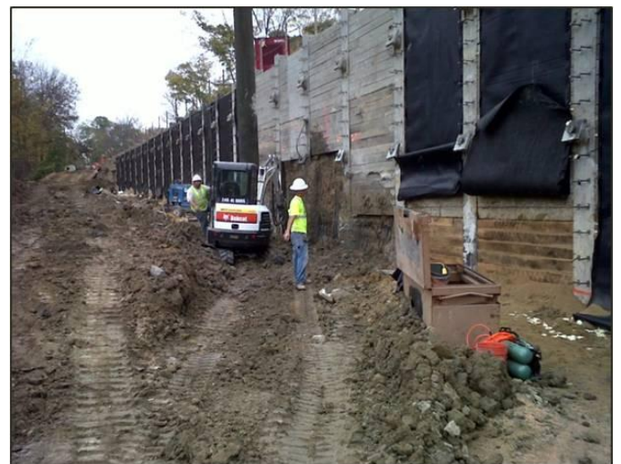
Fig. 23. Retaining Wall Drainage Installation
