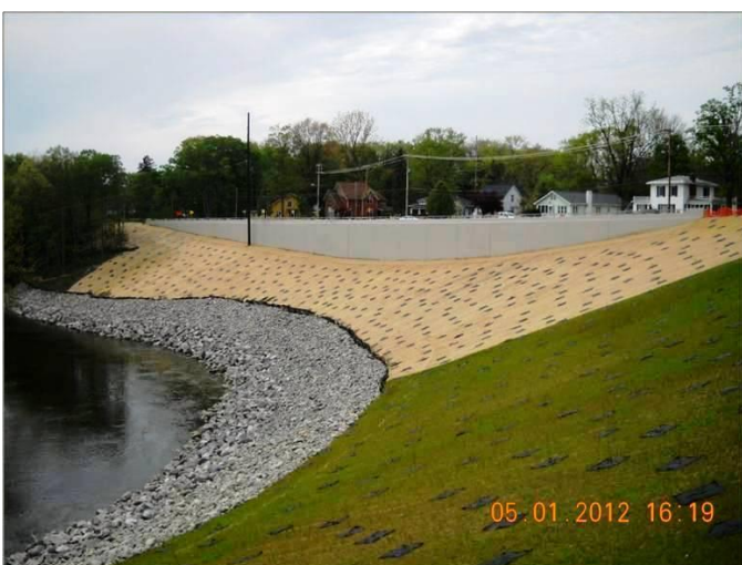
Fig. 25. Completed Project (Prior to Bareroot Planting)
