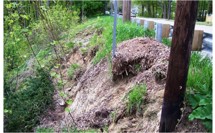
Fig. 3. Scarp Adjacent to M-222 (2009)
