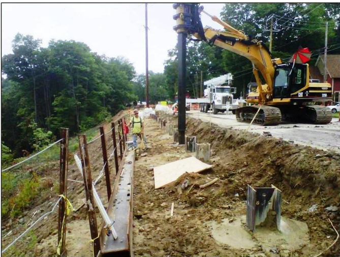
Fig. 18. Soldier Pile Installation
