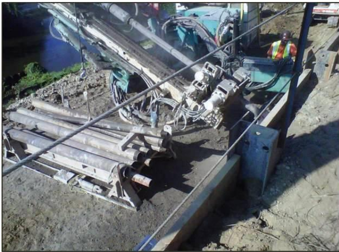
Fig. 20. Ground Anchor Installation
