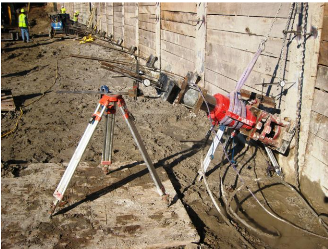
Fig. 21. Ground Anchor Stressing
