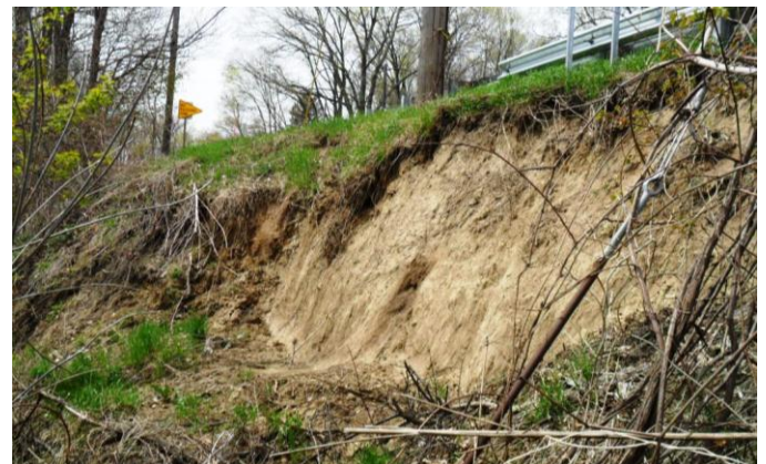
Fig. 4. Scarp Adjacent to M-222 (2011)
