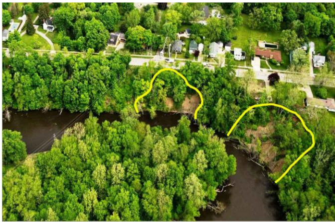
Fig. 7. Aerial View of Slope Instability (2011)
