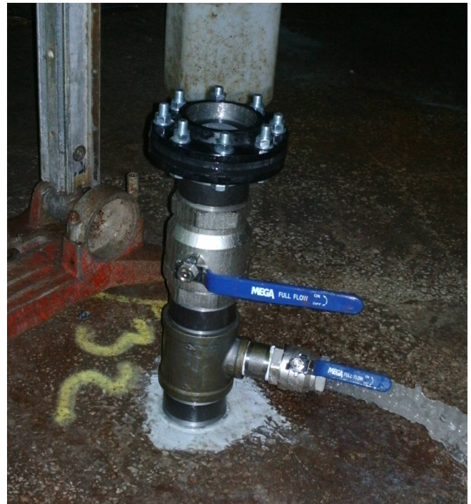
Fig. 12 – ‘Stuffing box’ installation
