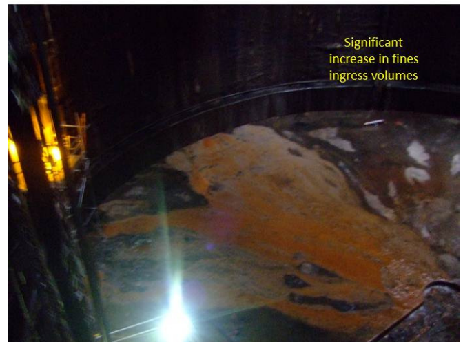
Fig. 3 – Notable increase in fines ingress volume between March 2008(a) and March 2009 (b)
