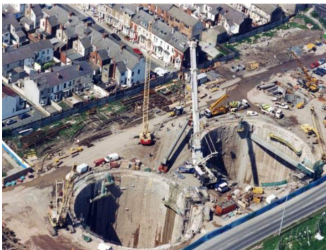
Fig.2- Aerial photograph of tanks during construction, 1999
