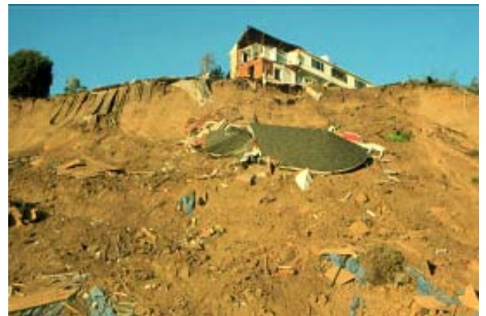
Fig. 3. Photograph of a house that was destroyed as a result of a slide at Pacific Palisades, by the Northridge, 1994, earthquake. ( http://pubs.usgs.gov/of/1996/ofr-96-0263 , 2006)
