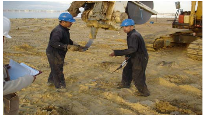
Fig. 12. Preparing PVD installation.
