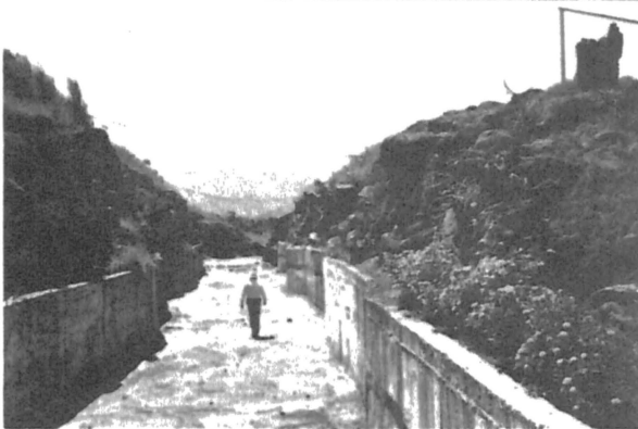
Fig. 13 View of Waste Weir After Lining.
