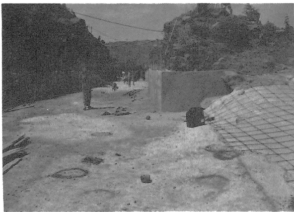
Fig. 14 Pointing of the Dam Rip Rap and Gunniting.
