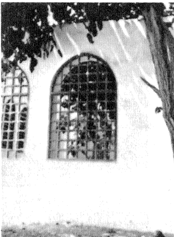
Fig. 13 Part of North Wall After Repair.
