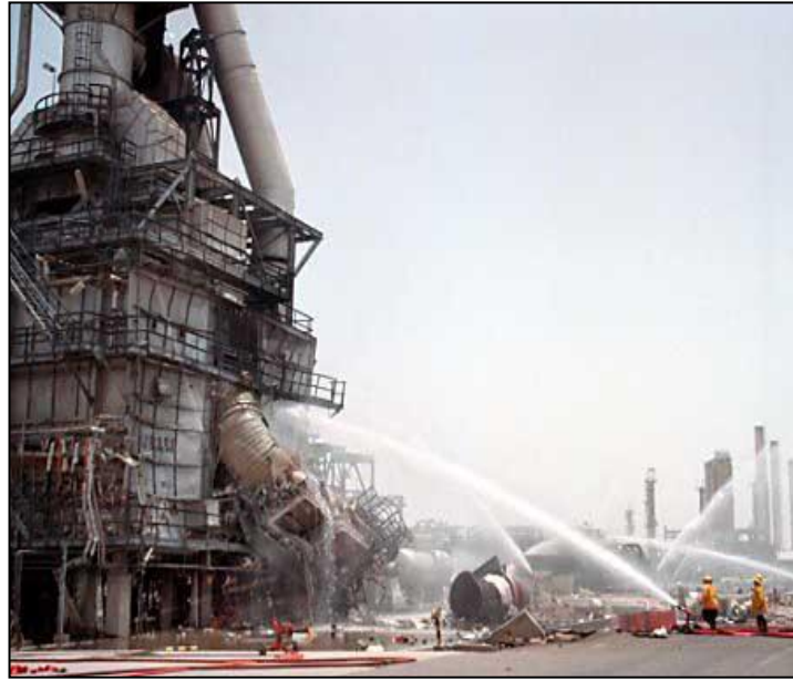
Figure 2. A Benzene unit destroyed during the explosion (KNPC, 2014)
