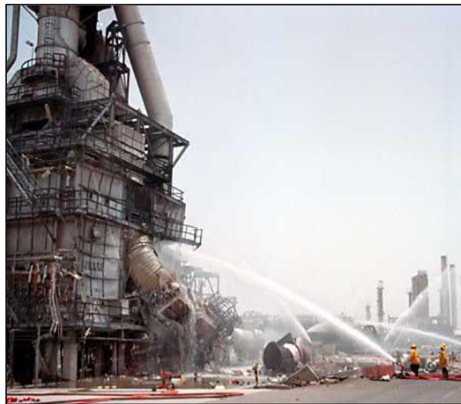
Figure 9. One of the Benzene units destroyed during the explosion (KNPC, 2014)
