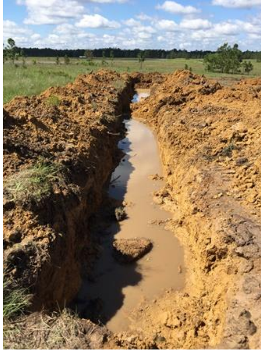
Figure 18: Drainage Ditch from Section 1
