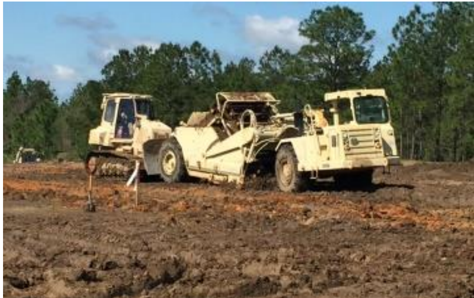
Figure 19: 613B Scraper Receives T5 Dozer Push Assist
