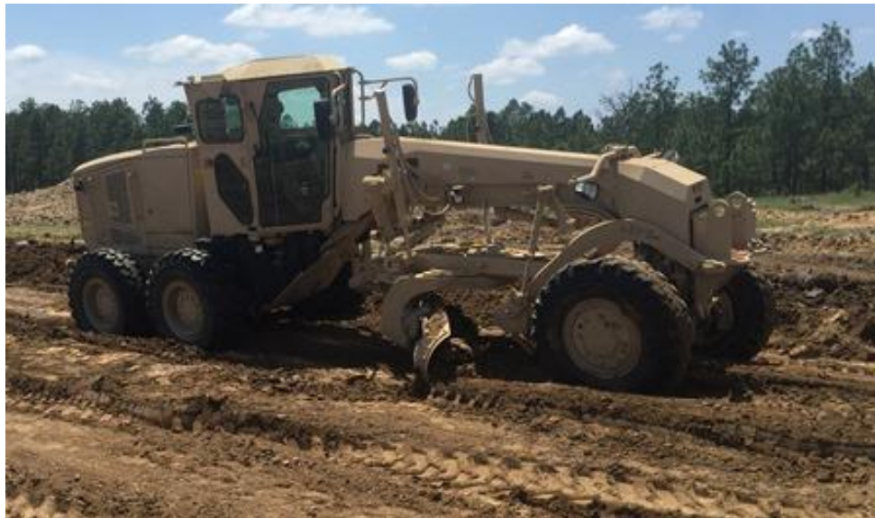
Figure 24: Grader Excavation Work
