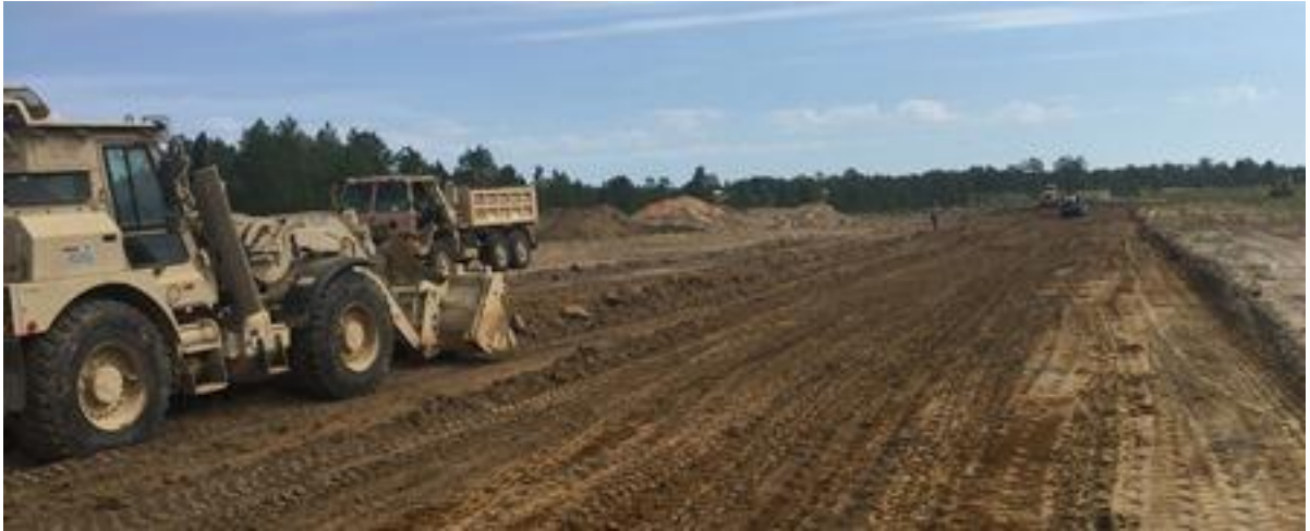
Figure 25: FLS Berry Windrow Excavation
