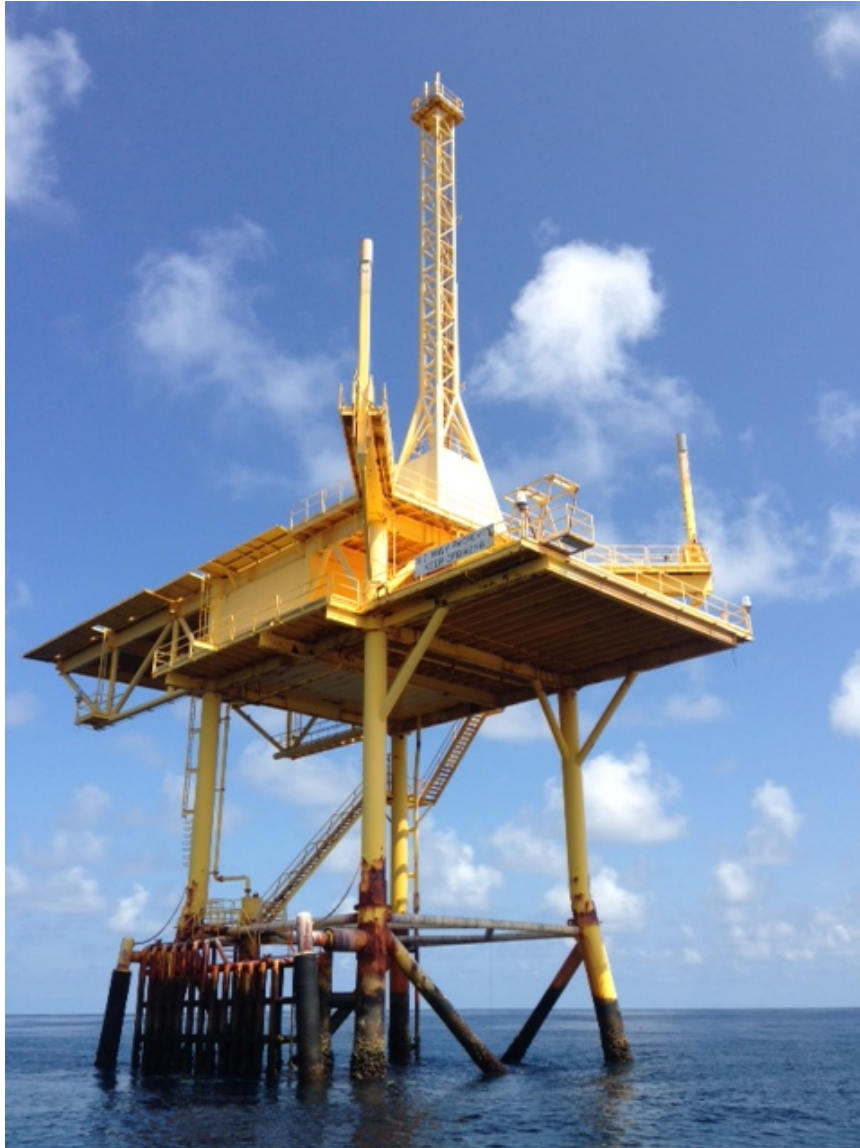
Figure 2.3: Abandoned Navy Tower R2 (31°22'30"N, 80°34'01"W) off the coast of Georgia. All three Navy Towers used in this study (R2, M2R6, and R8) are similar in design and size (Photo credit to Chris Briand).
