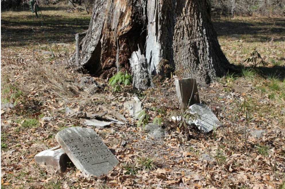
Figure 35: Mont Repose Cemetery Gravestone Damage (a)
