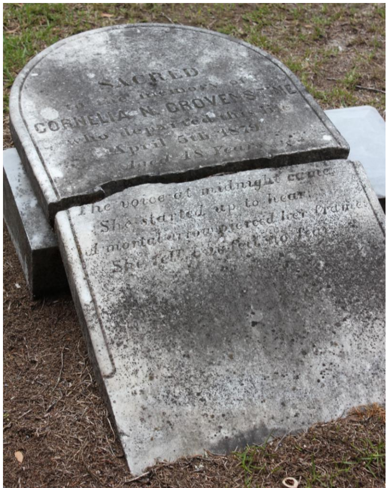
Figure 48: Ebenezer Cemetery Gravestone Damage (i)
