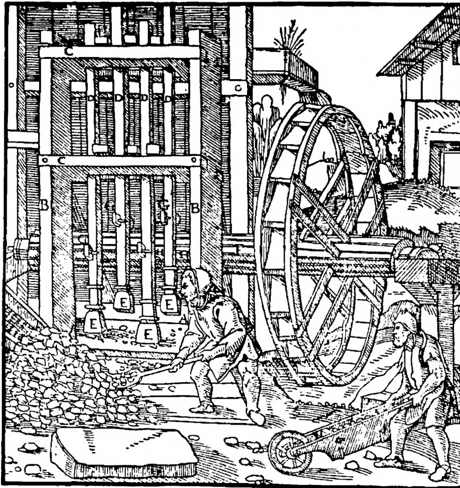
A—MORTAR. B—UPRIGHT POSTS. C—CROSS-BEAMS. D—STAMPS. E—THEIR HEADS F—AXLE (CAM-SHAFT). G—TOOTH OF THE STAMP (TAPPET). H—TEETH OF AXLE (CAMs).
