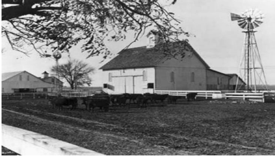
Figure 7: American windmill for water pumping (US Department of Agriculture)
