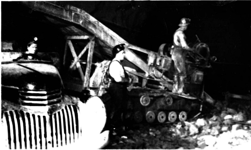
Fig. 2 Mobile electric slusher ramp, mounting a 20 h.p. 3-drum electric hoist which pulls a 42-inch scraper, loading into a two-ton Chevrolet dump truck converted to diesel.
