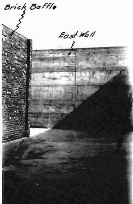
Interior of Sedimentation Basin
