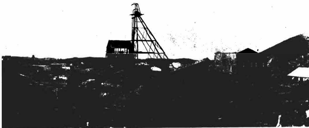
THE SHAFT — LOOKING NORTH
