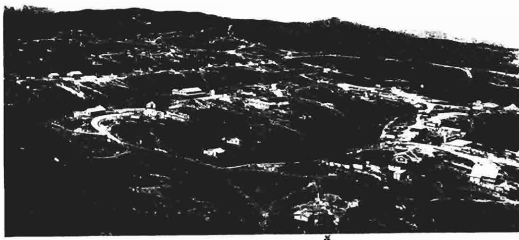
MATANAMBRE - LOOKING WEST Substation in Central Foreground
