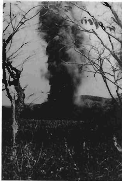
500-lb Refraction Shot in Mud Hole. Spanish America.
