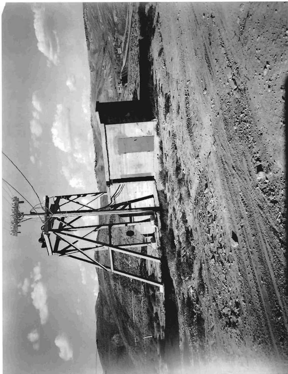
Number seven fan house with head frame
