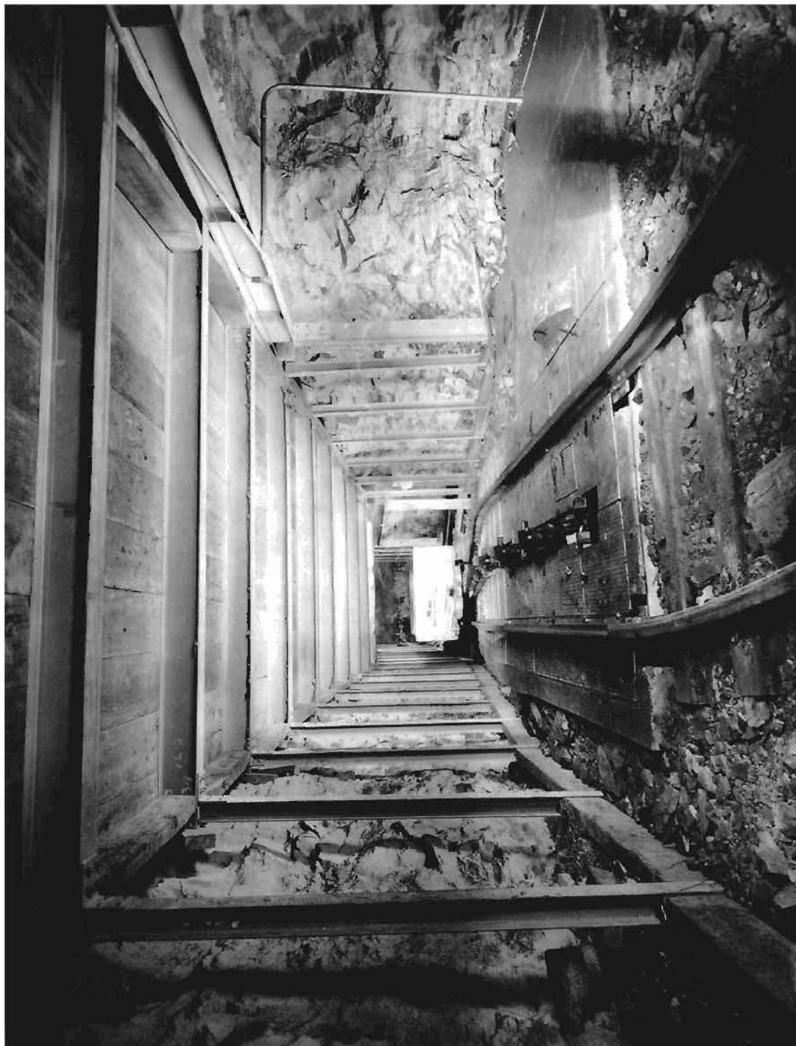
Car haul number seven seam--also showing steel sets and Redwood lagging.
