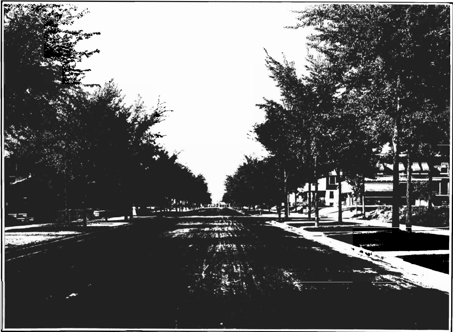
GLADSTONE BOULEVARD-Showing standard boulevard construction.
