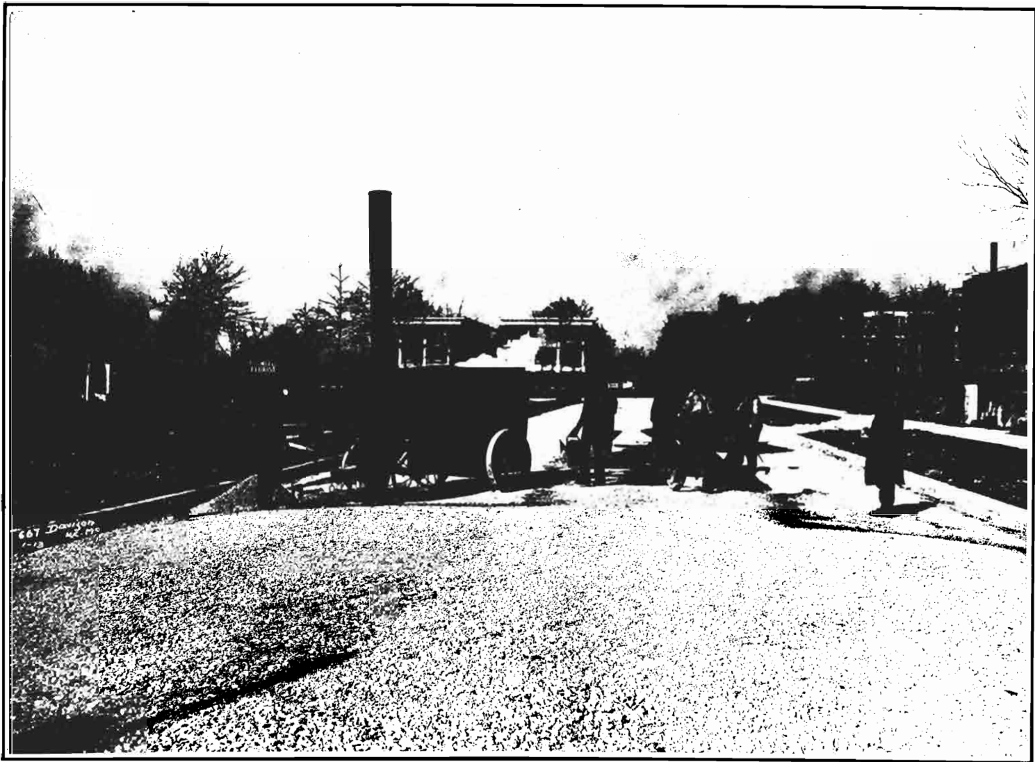
THE PASEO-Applying asphaltic cement.
