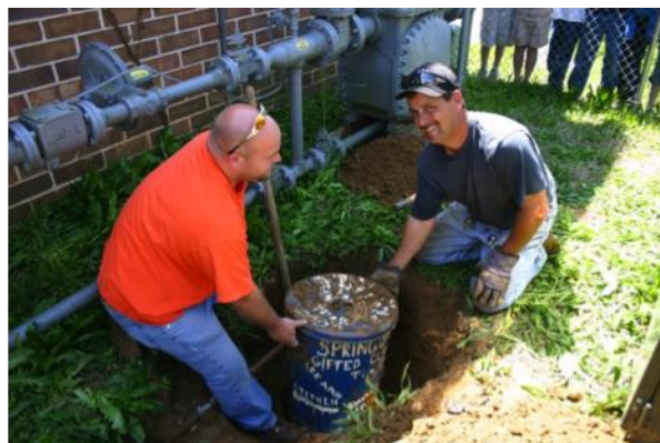
Figure 4. Workers remove capsule from the ground
