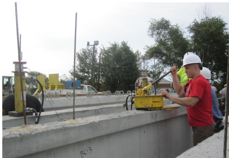
Figure 5.25 Strands being tested using pull-out test.
