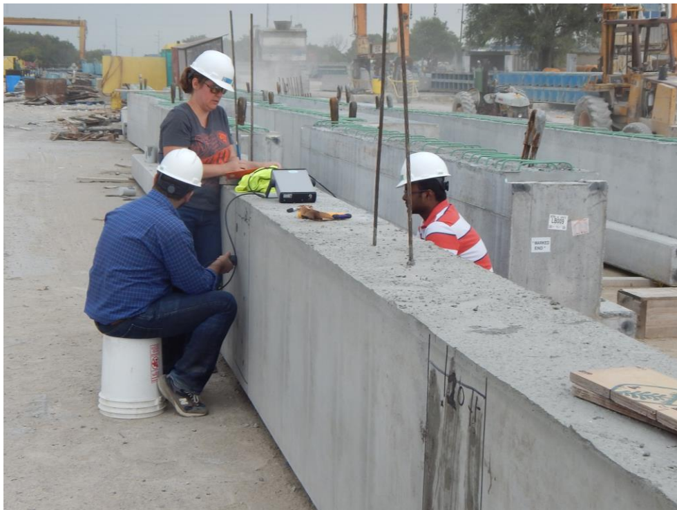
Figure 5.21 On-site UPV testing on beam.
