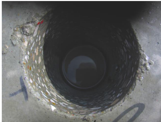
Figure 5.17 Drilled core in beam.
