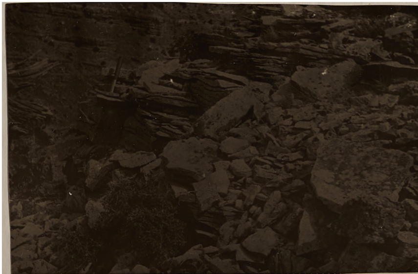
Plate 20 Facing North. Slabby dolomite beds overlying Madison Limestone at Little Popo Agie River measured section location. SW \frac{1}{4} Sec. 14, T31N, R 99 W.
