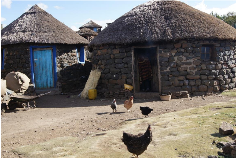
FIGURE 2 A man enters his rural Basotho home. The bundle of stalks on the side of the house will be used to repair the roof.
