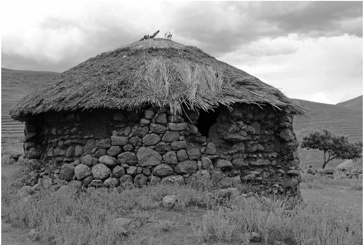
Figure 6: ‘M’e Masello’s house, which has been unoccupied since 2010; 2015.
