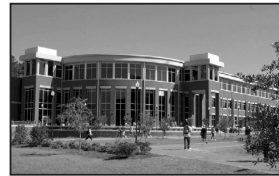
The College of Information Technology building
